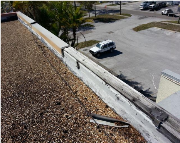
Missing and damaged cap flashing at the far west side of the roof
