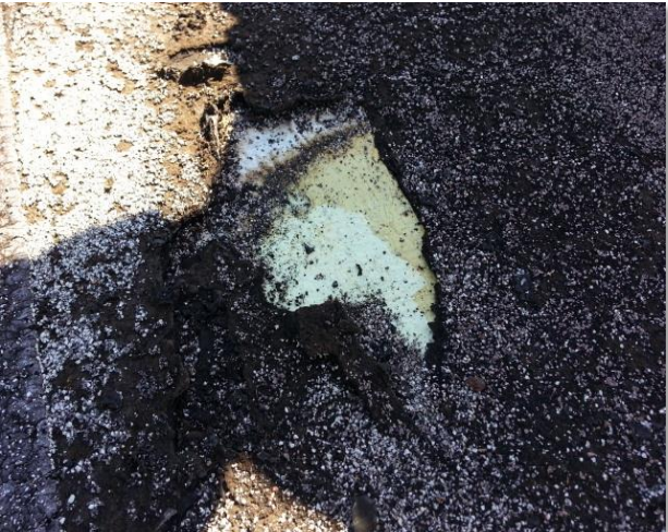
Old membrane has completely worn away
