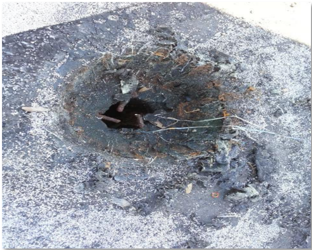
Roof drains are badly deteriorated
