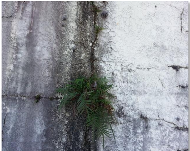
Heavy plant growth and algae on the north wall indicates extensive moisture intrusion
