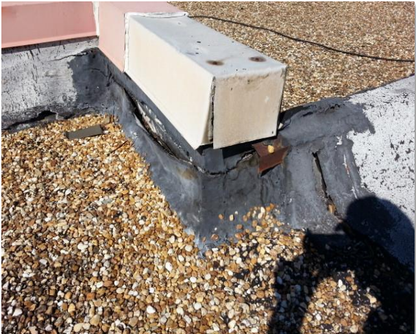
Deteriorated and open membrane at the west side parapet walls
