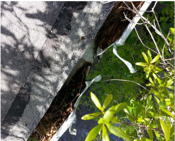
The gutter system needs to be replaced at this time
