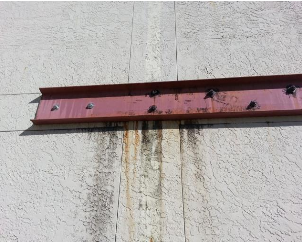
Steel ledger on the south wall should be removed
