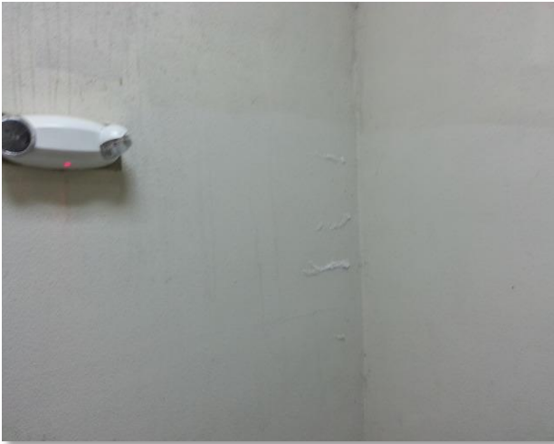
Water intrusion through walls
