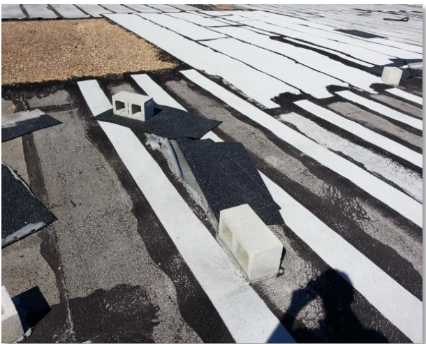
Example of widespread and poorly installed patches to the roof
