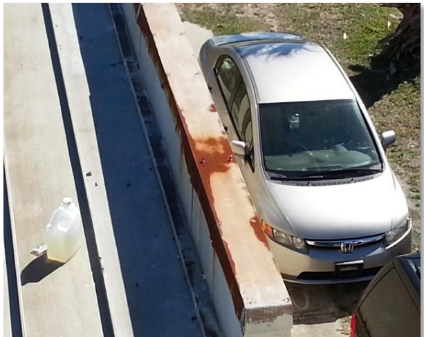
Deterioration to the accessory structure parapet cap flashing
