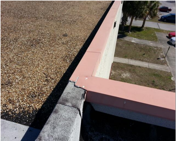
Poorly integrated cap flashing and membrane
