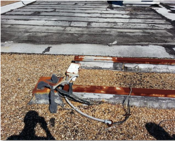
Exposed wires on the roof
