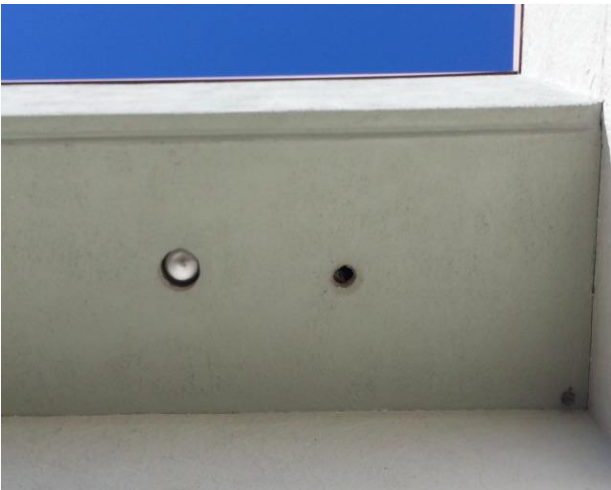
Poorly sealed soffit lighting
