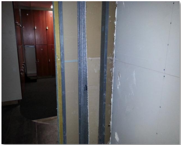
Example of unfinished interior wall framing
