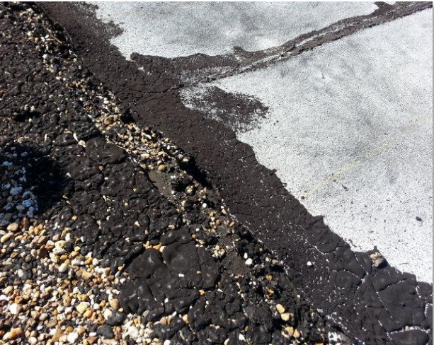
Example of many lifting sections of mod. bit.
