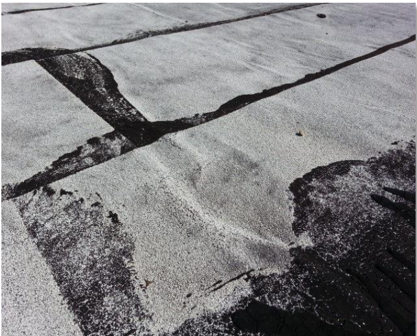
Very uneven roof deck
