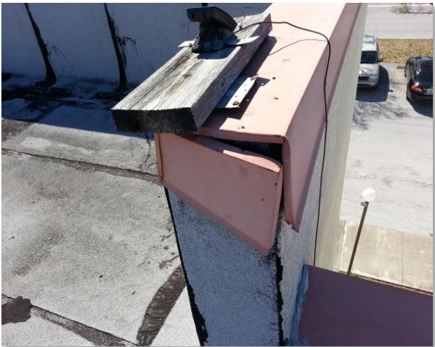
Loose cap flashing at the west side over the front entry
