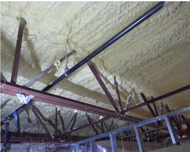
Foam insulation in the west area of the building
