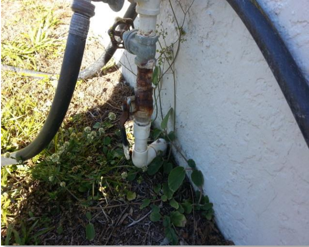
Main water shut-off valve
