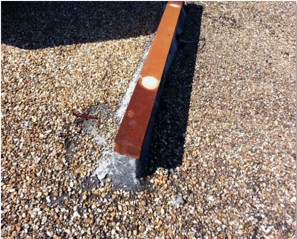
Example of badly rusted flashings
