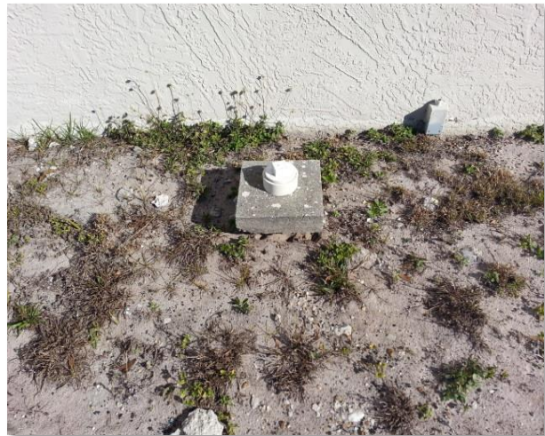
Example of about 4" of soil loss around the building
