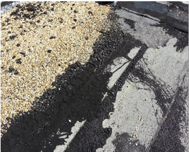
Deteriorated and crude intersection of gravel and older mod. bit. roofs
