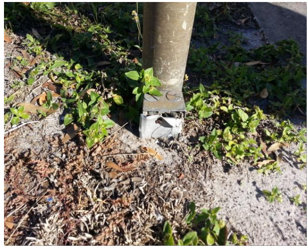
Damaged junction boxes at exterior lighting
