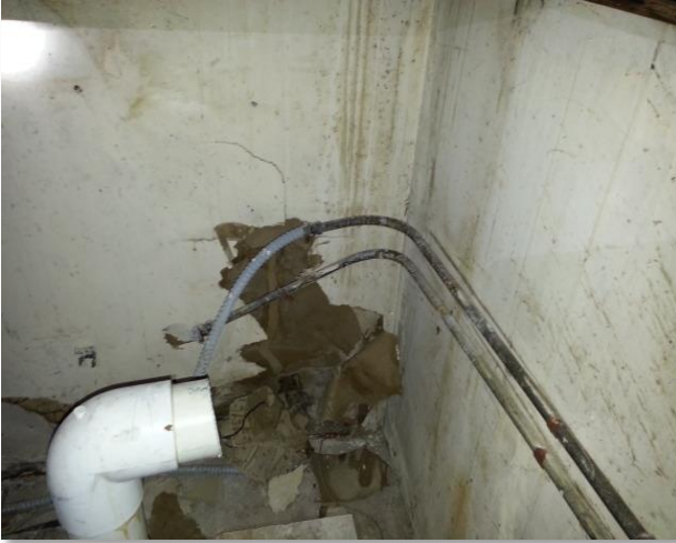
Water and fungal damage to the wall in the ladies Jacuzzi equipment room
