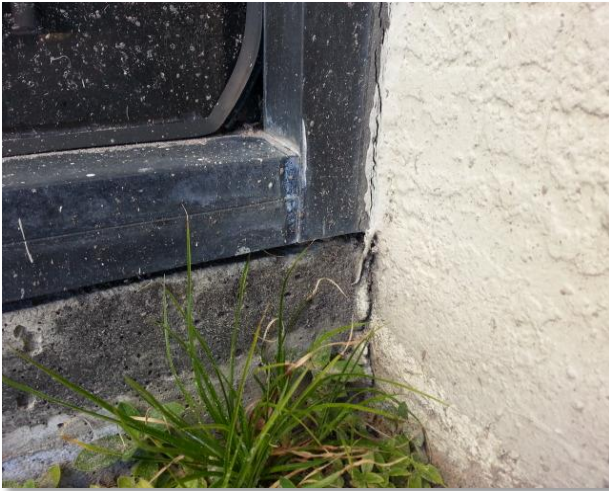
Deteriorated sealant at windows
