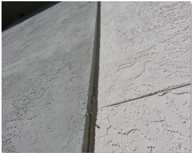
EIFS panels are poorly sealed and are prone to water intrusion
