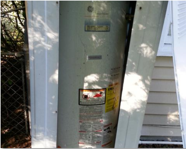
Main water shut-off valve
