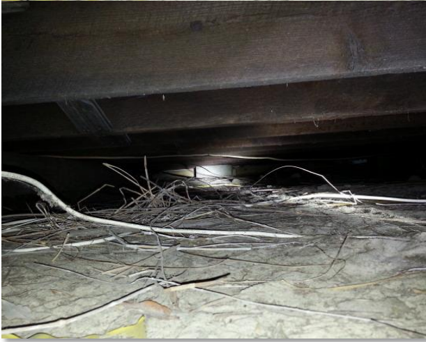
Under floor view
