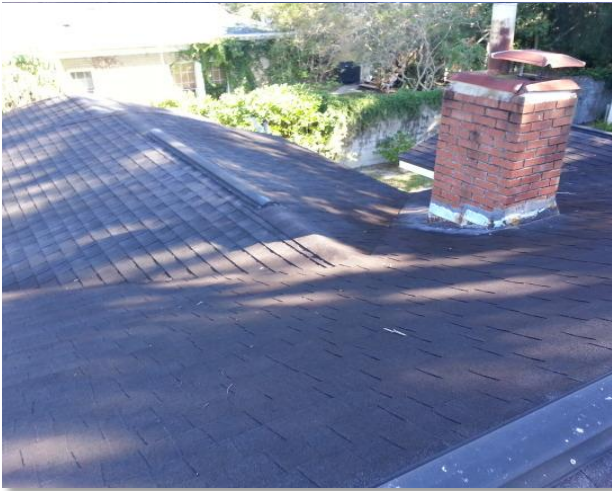
General view of roof front
