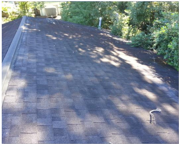
General view of roof rear
