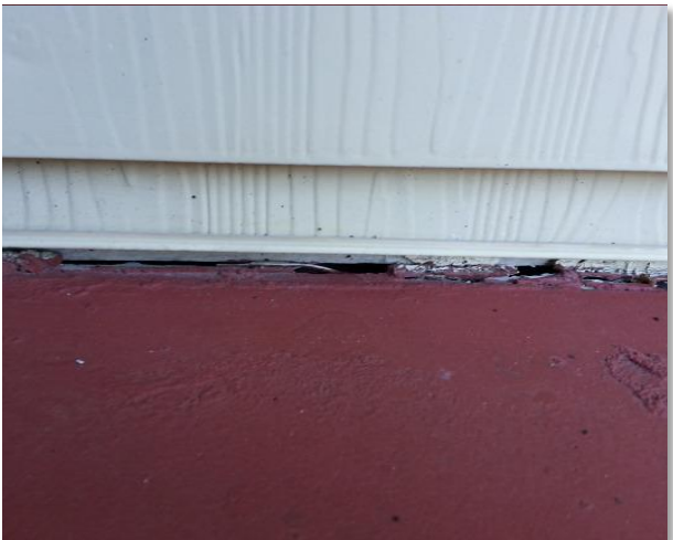
Seal intersection of front porch and house
