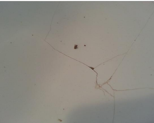
Damaged apartment sink
