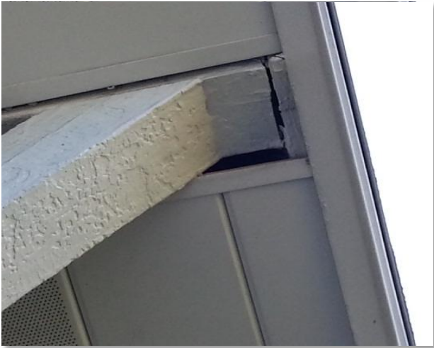
Seal around trim and soffits
